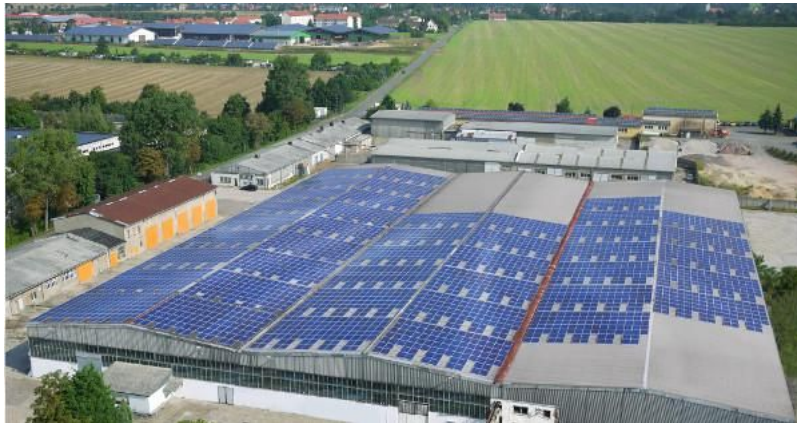
Solardach in Dahlen
