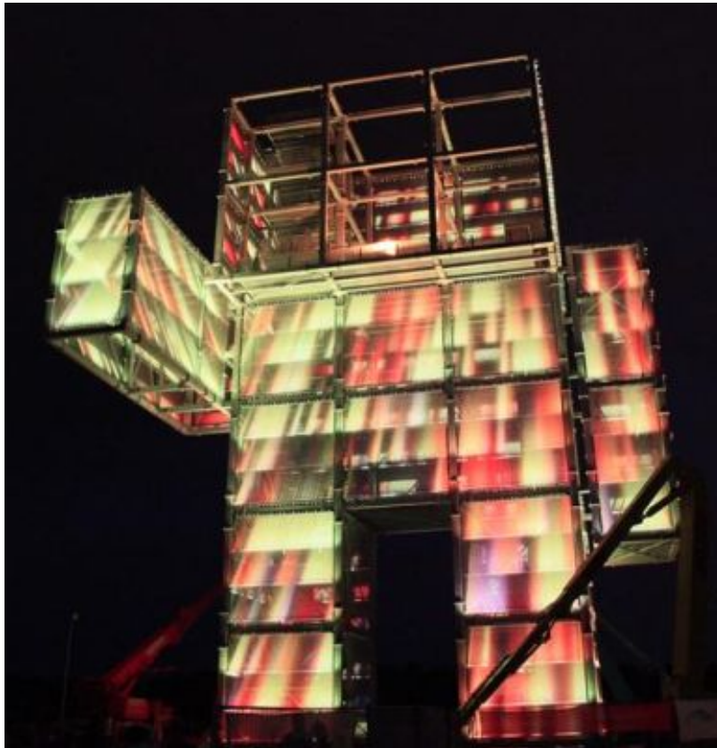
Indemann ©ag4 media facade GmbH
